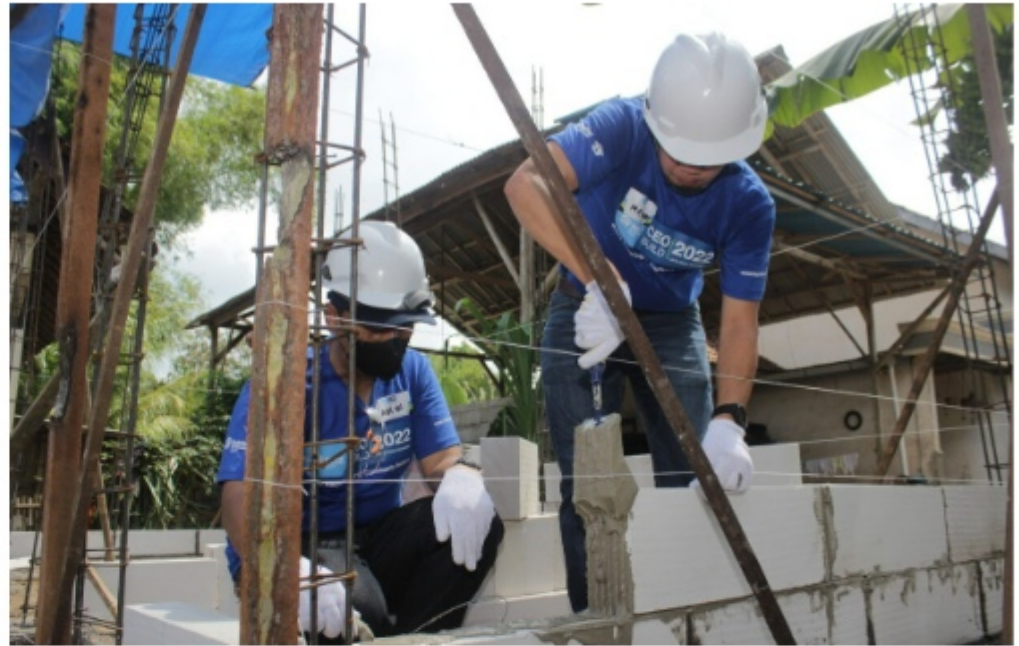
Volunteers at the CEO Build 2022 in Banyuwangi.
