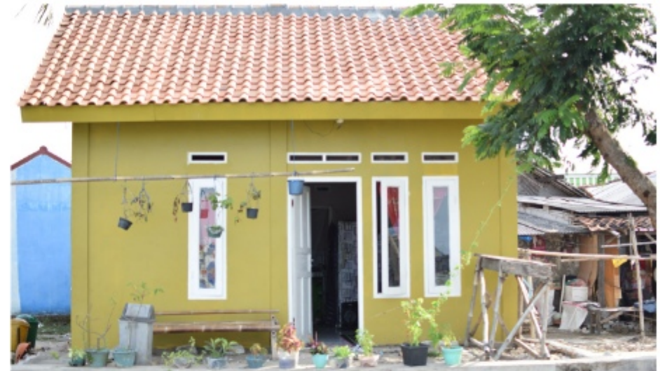
The house of Tisah after reconstruction. Sumber Foto: Comm Habitat Indonesia
