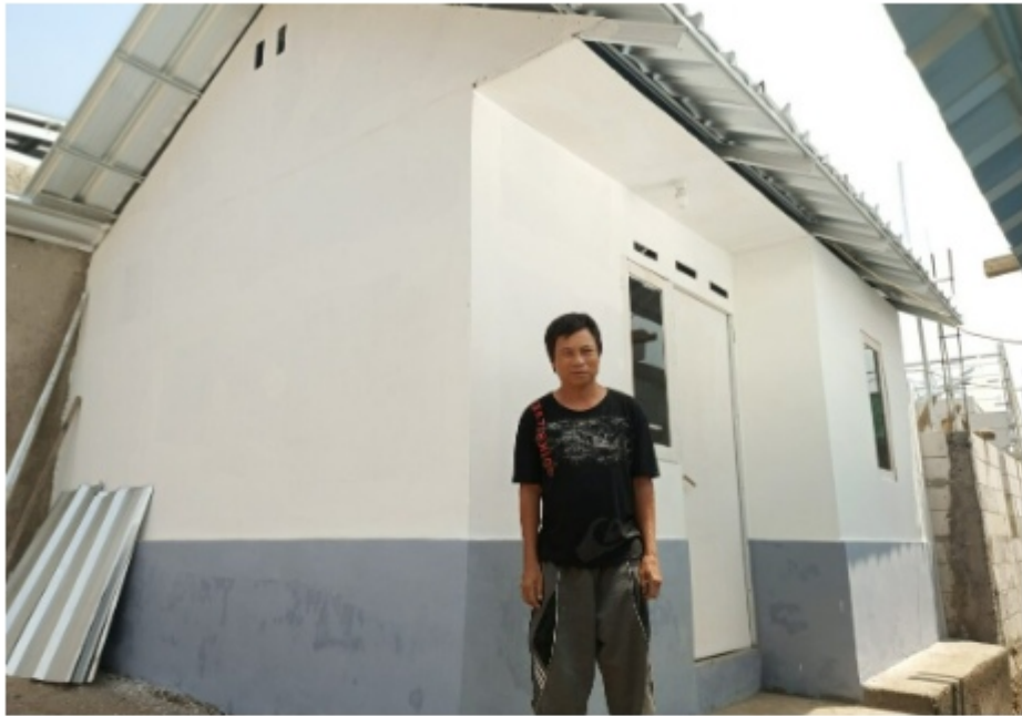
Temporary Housing in Cianjur.
